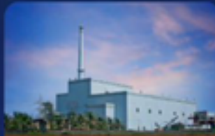
TAPS - 162 / Tarapur Atomic Power Station (Tarapur, Maharashtra)
