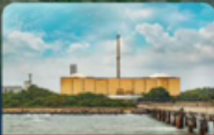
MAPS - 162 / Madras Atomic Power Station (Kalpakkam, Tamil Nadu)
