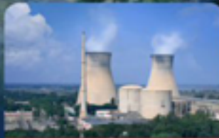
NAPS - 162 / Narora Atomic Power Station (Narora, Uttar Pradesh)
