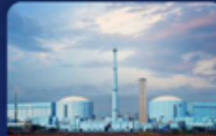
TAPS - 364 / Tarapur Atomic Power Station (Tarapur, Maharashtra)
