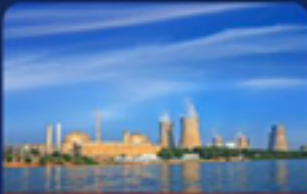
RAPS - 166 / Rajasthan Atomic Power Station (Rawatkhata, Rajasthan)
